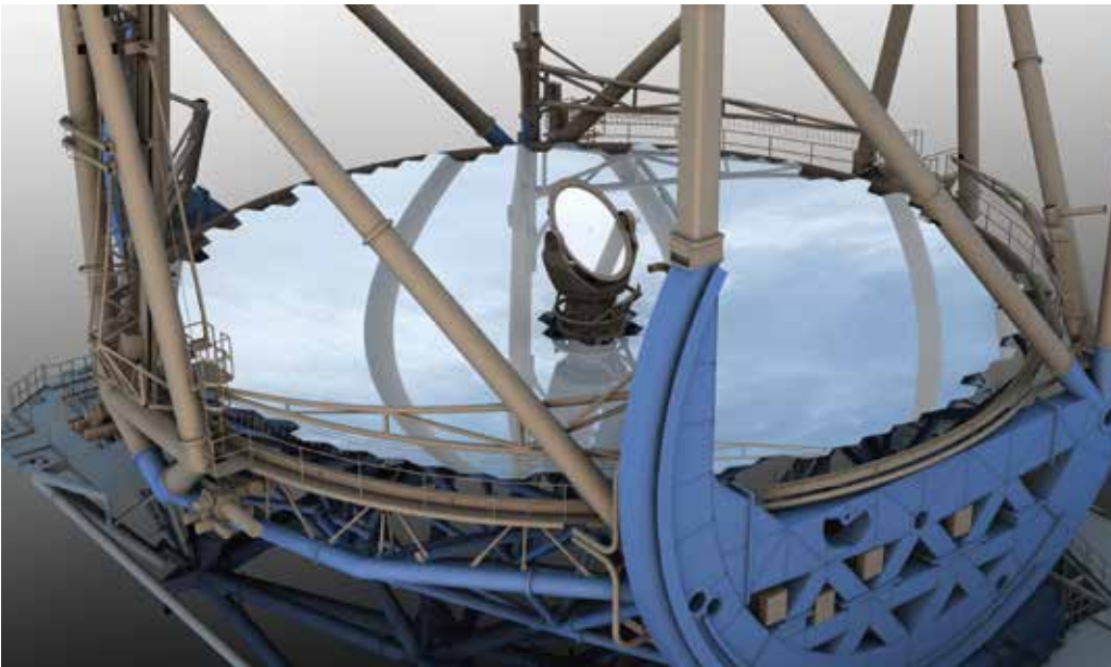
30 meter primary mirror comprised of 492 segment mirrors. Segment mirrors 1.44 m in length across corners are laid out with 2.5 mm of spacing.
